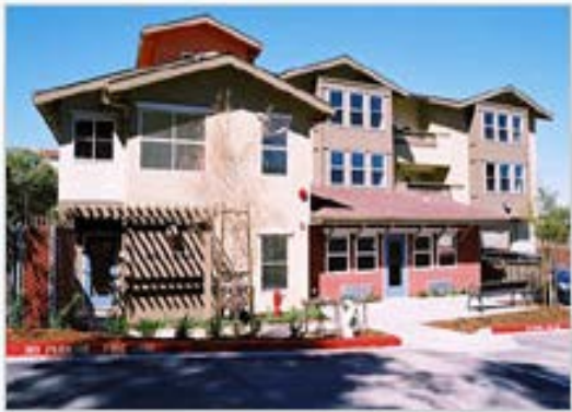
Cedar Street Apartments - Approved in 2009 (5 units)
