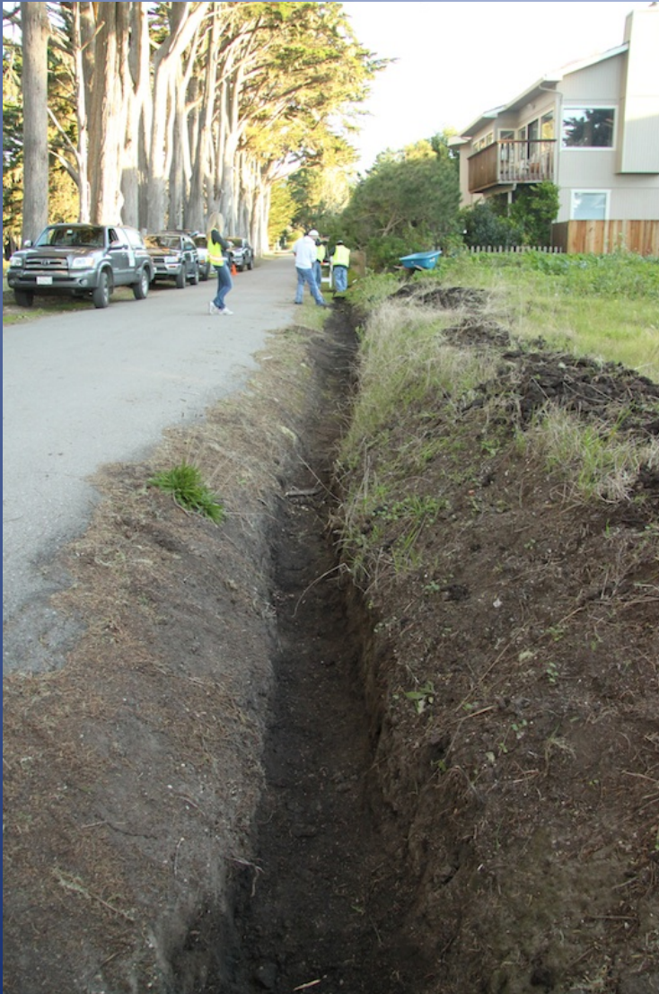
Cypress Ave Trench
