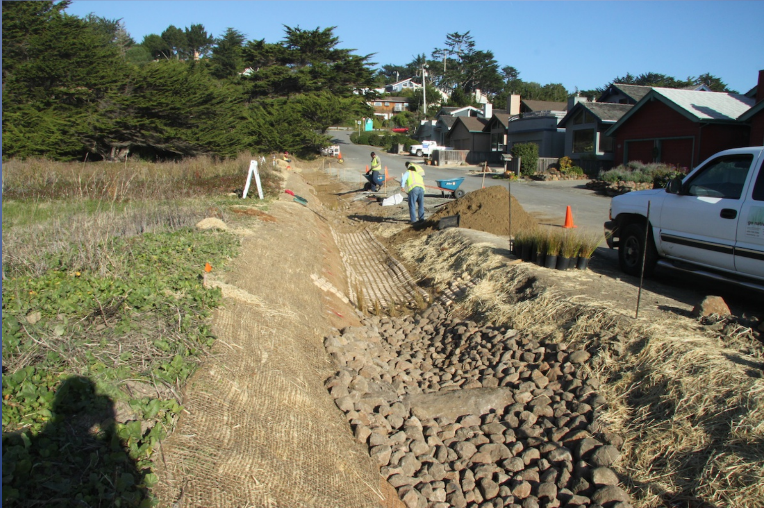
Finished rock weirs and paver installation at Juliana Swale
