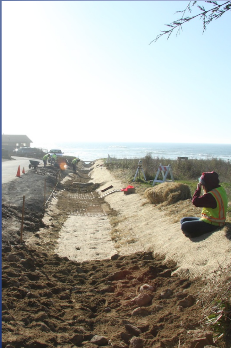
Finish Work at Juliana
