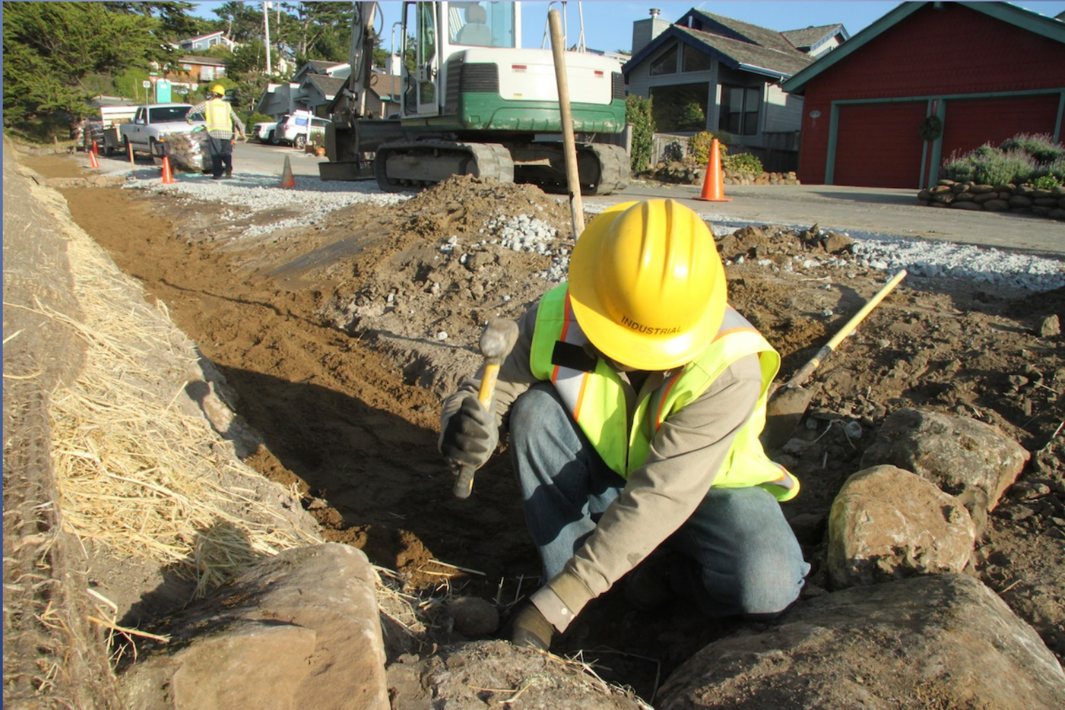
Construction of rock weirs at Juliana Swale
