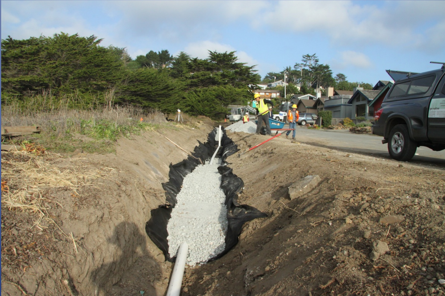
Installation of filter fabric, drain rock and rain pipe at Juliana Swale
