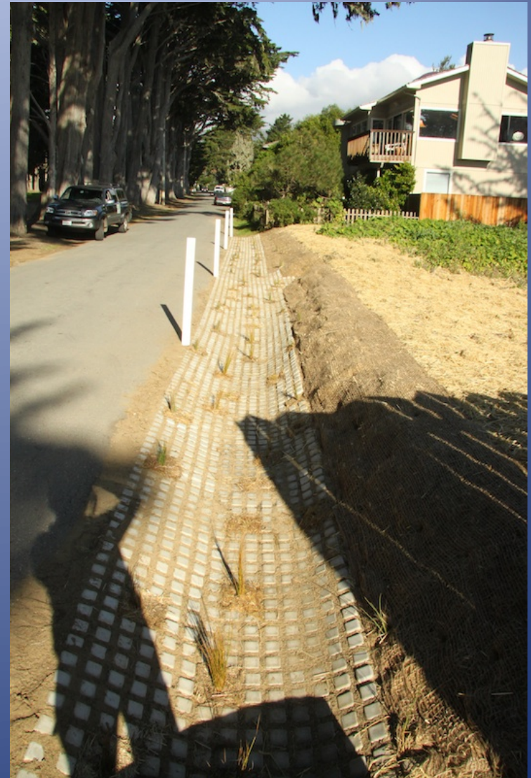
Completed Cypress Swale
