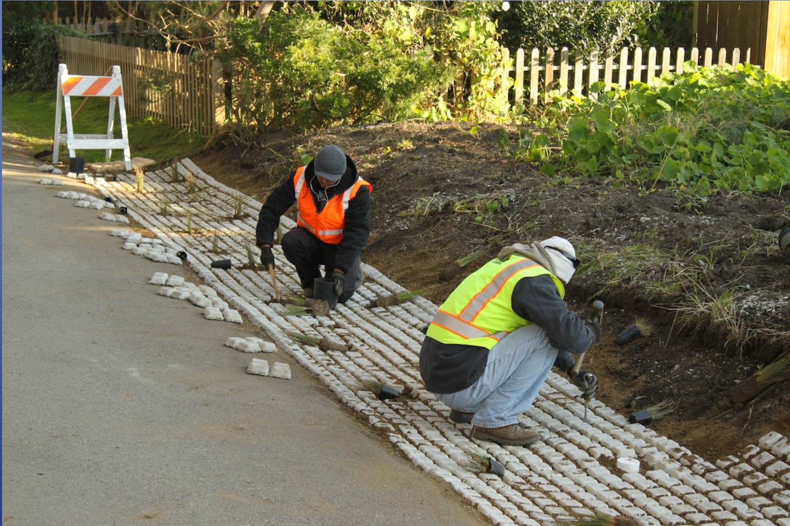
Installation of Native Plants at Cypress Swale
