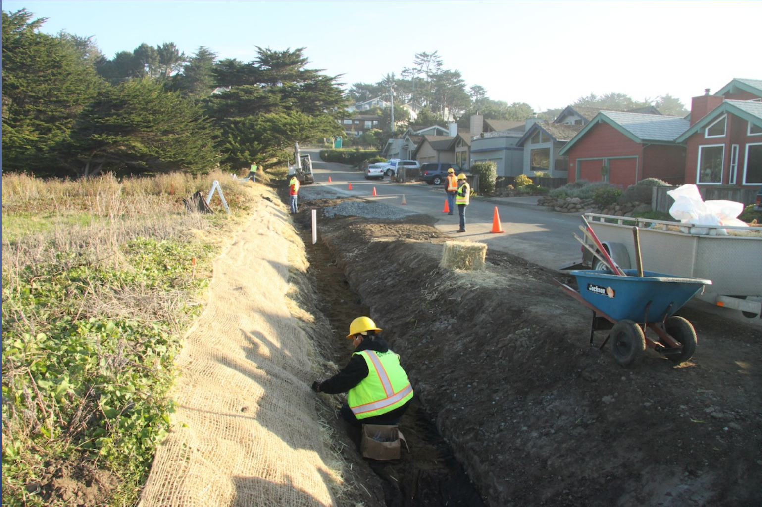
Installation of biosoil and erosion control material at Juliana Swale
