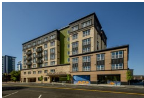
Arroyo Green Senior Housing 6 Units
